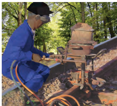
Figure 3.11 Thermit process for joining railway tracks
